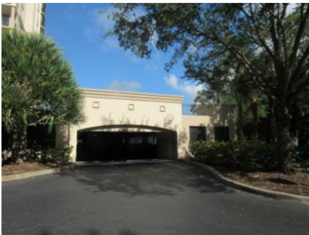
View of typical asphaltic pavement located throughout the subject property.
