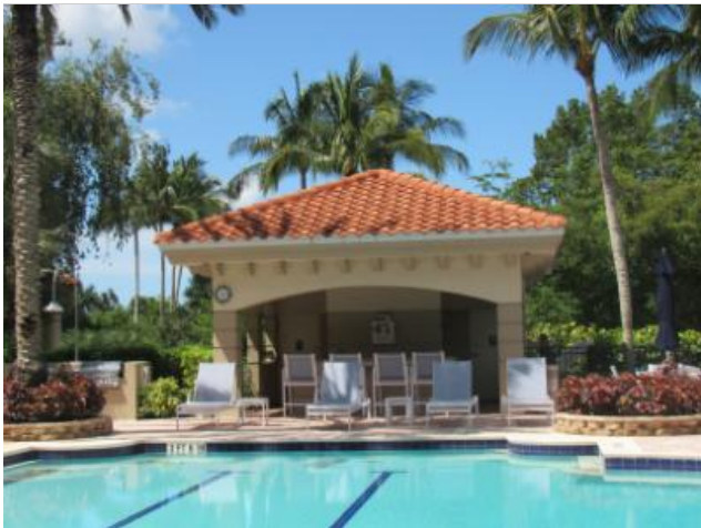
View of subject pool pavilion clay tile roofing system.
