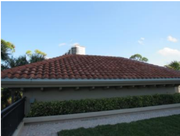
View of subject mechanical building roofing system.
