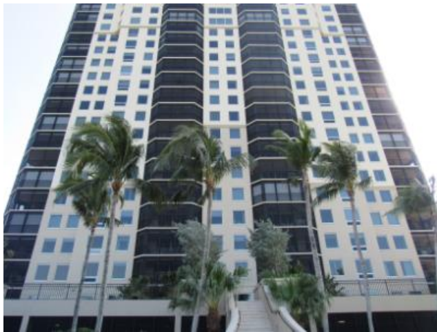
Overview of subject unit balcony screen enclosures and railings.
