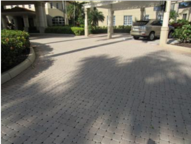
View of subject roadway and/or parking concrete pavers.
