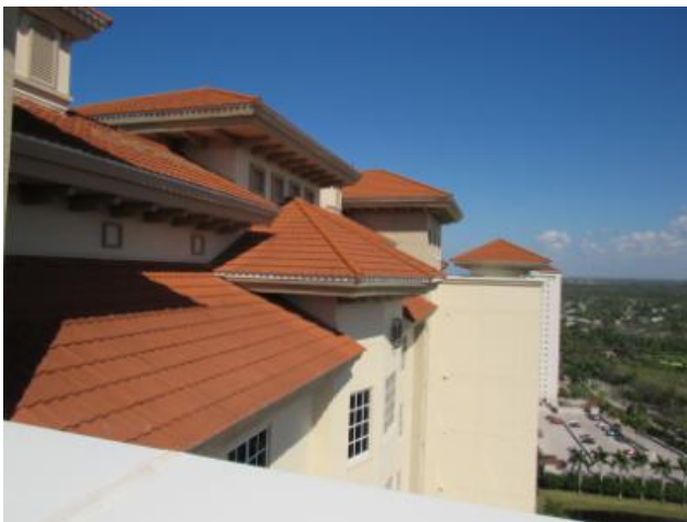
Subject tower sloped roofing system observed during our site inspection.
