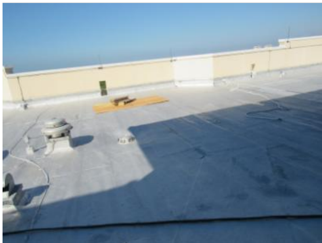
Subject tower flat roofing system observed during our site inspection.
