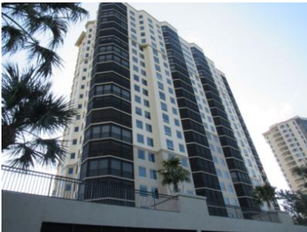
Overview of subject building exterior observed during our site inspection.
